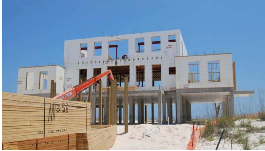
A beachfront home that is built to withstand hurricanes. The ICF home is built on stilts in the Gulf Coast.
