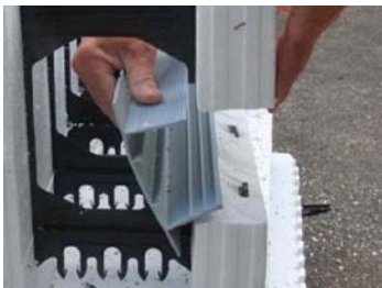
Installing a channel in the block.
