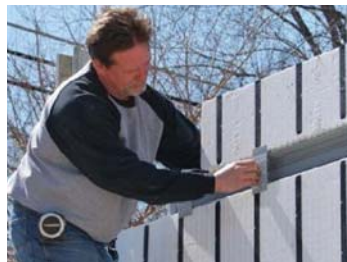
Infield installation of the e-channel.
