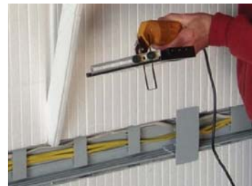
Removing foam to install remote power.
